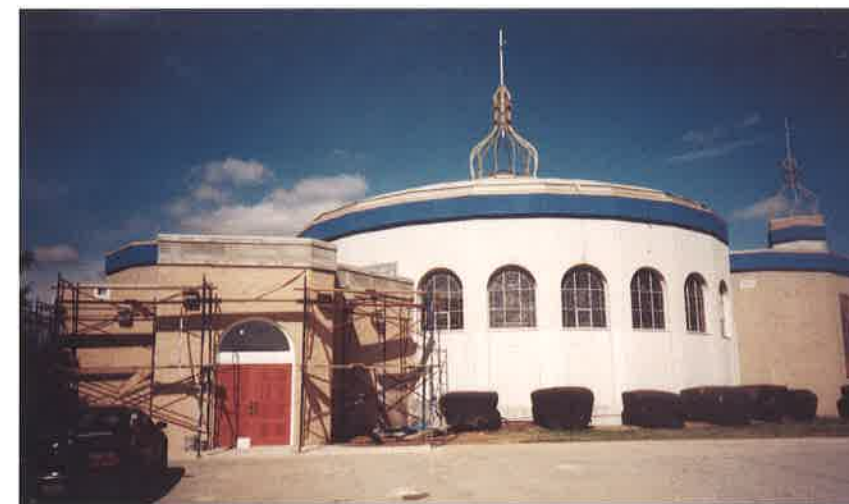
Building the new addition.
